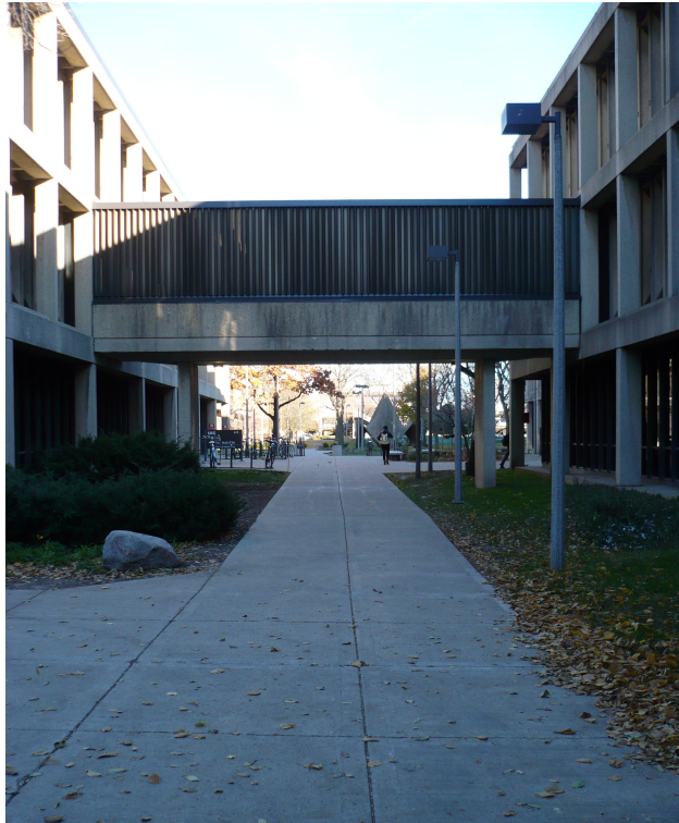
Only a few minor, smaller walkways survived the Coffey-led renovations.
