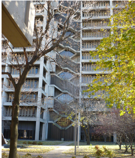
The Science and Engineering Offices Building features concrete scissor staircases.
