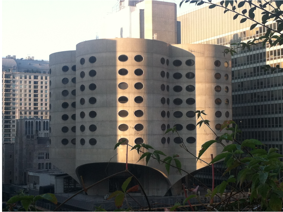
Preservationists argued Prentice’s cantilevered shell was among the many features that spoke to its structural importance.
